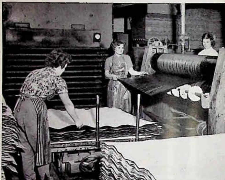
FIG. 2/5. Phenolic resin glueing of veneers in Finland for tropical plywood.
